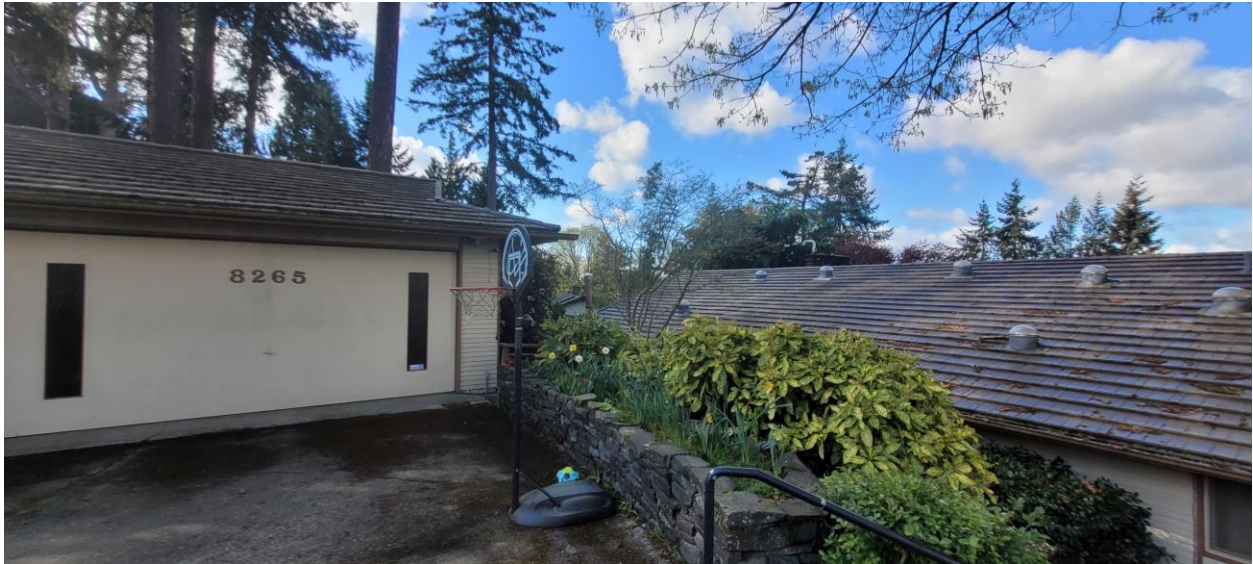
Photo 1: Existing garage/driveway in relationship to house
